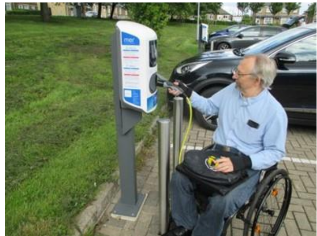
Image 2: Wheelchair user accessing a front-facing charging device mounted at vehicle bay level with bollard protection in front of kerb.
